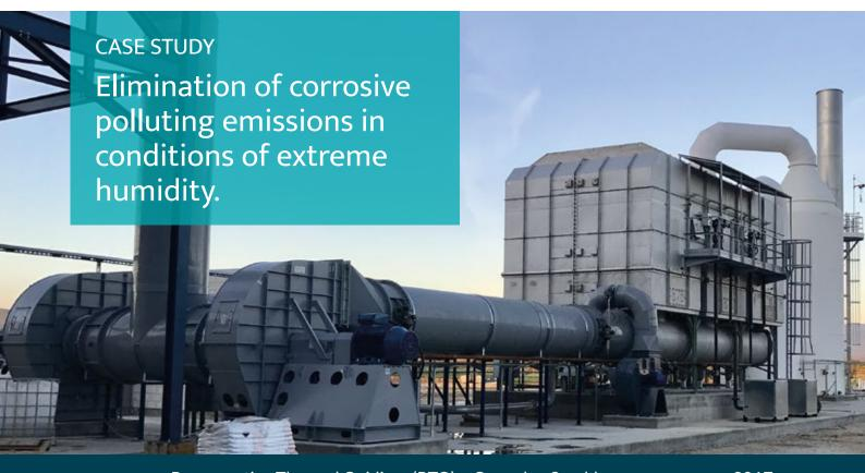
Equipment: Regenerative Thermal Oxidizer (RTO) + Quench + Scrubber. Installation: 2017
